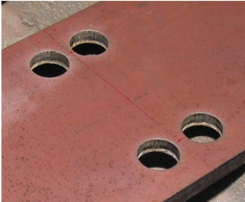
Figure 4-1 Phase 1 of making slotted holes
